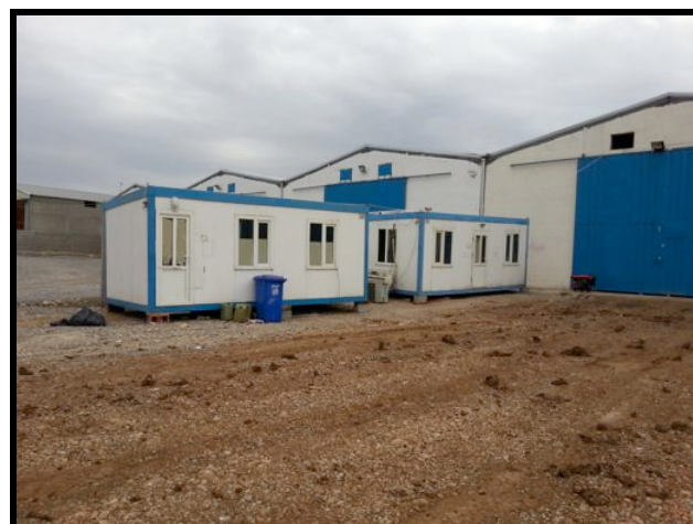
Security staff and generators are provided with some warehouses
