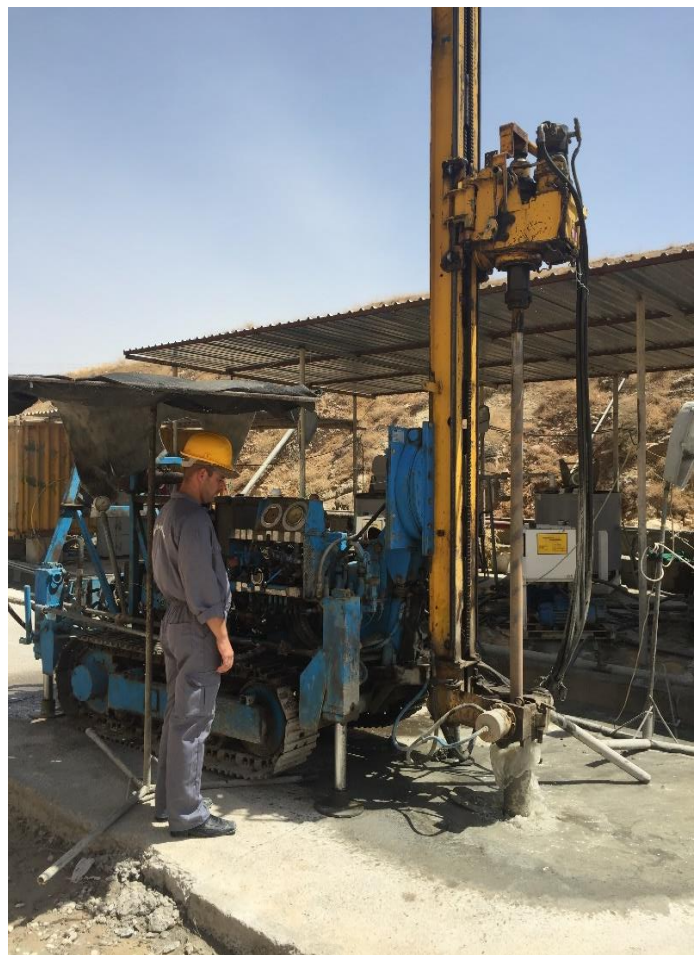
Figure 3: Grouting along the side of the Spillway Chute
